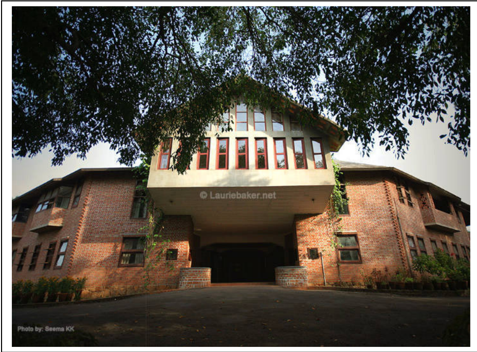
Centre for Development Studies ( Trivandrum ) Laurie Baker Construction Approx Cost : 700 / Sq Ft
